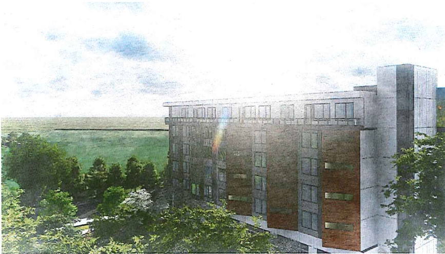
EAST ELEVATION - VIEW FROM HILL
